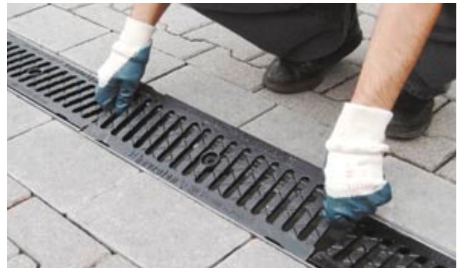
1. PUT SIDE-LOCK IN PLACE
