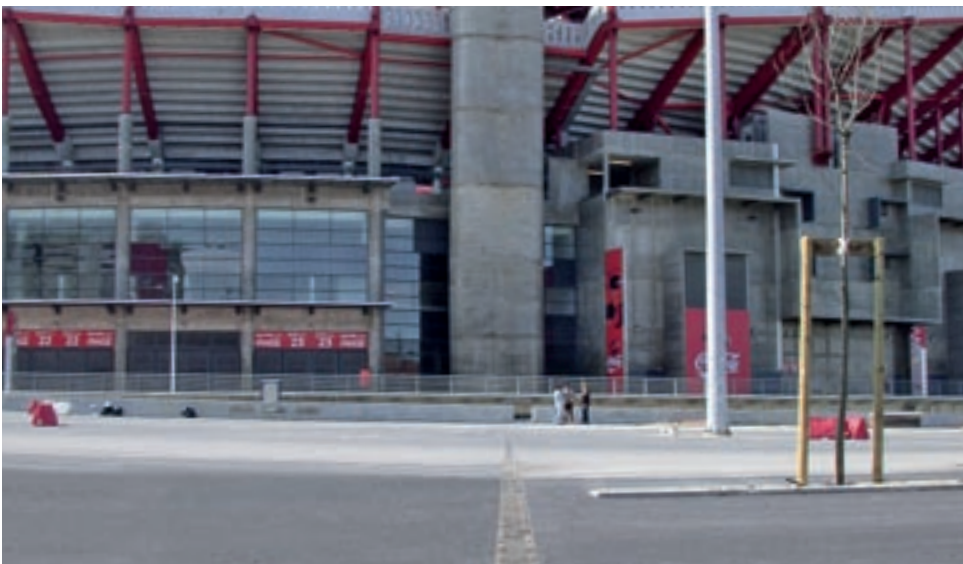
FASERFIX SUPER KS 100 Channels in front of the Estádio Da Luz in Lisbon
